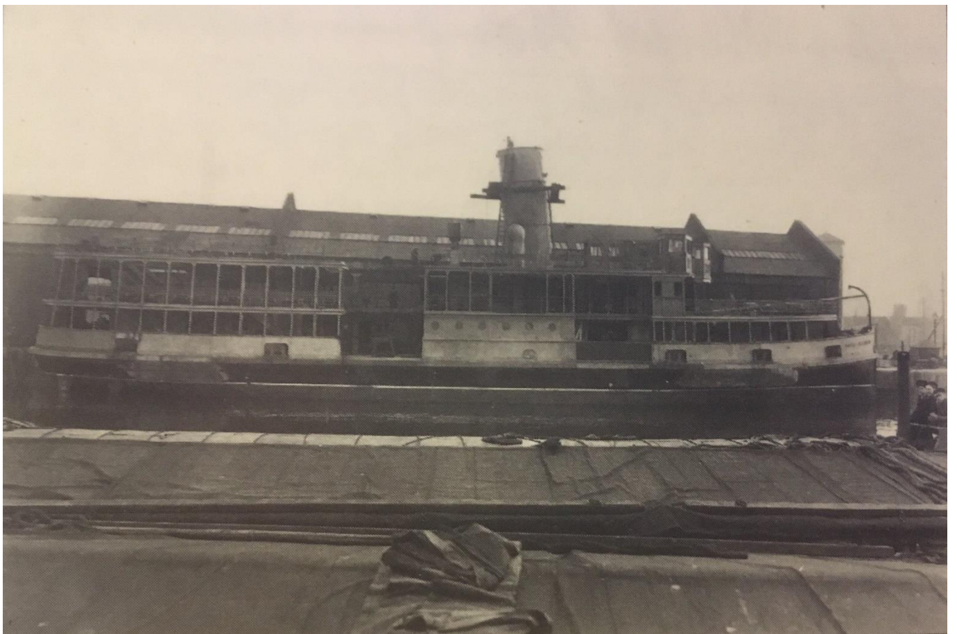
Re-floated, under repair
